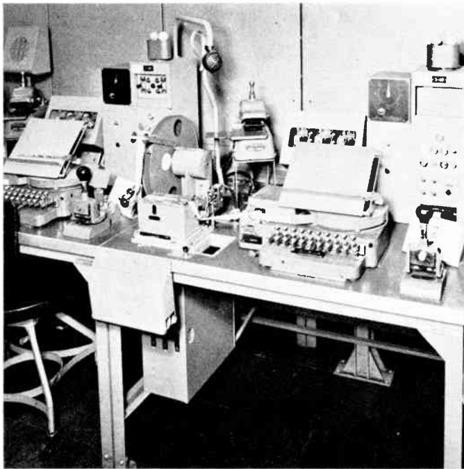
Figure 41. Local operator's sending position
