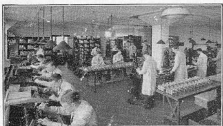
A Section of the Wiring Department
