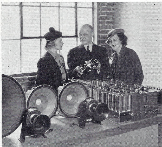
The 40 Tube Chassis, 18-in. Bass Speaker, Two 12-in. Mid Frequency, and Two High Frequency Speakers.
