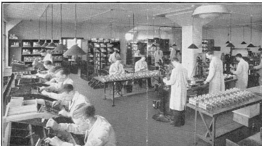
General View of Assembling and Wiring Department
