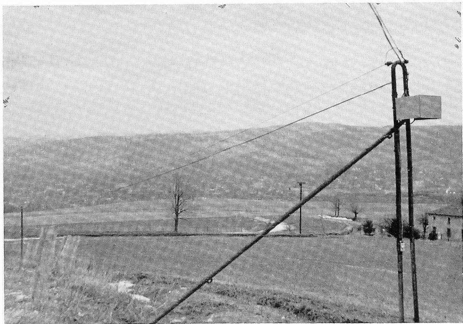
Fig. 5. Distribution Amplifier Mounted on Utility Pole. (Photograph by courtesy of Taco Antenna Co.)
