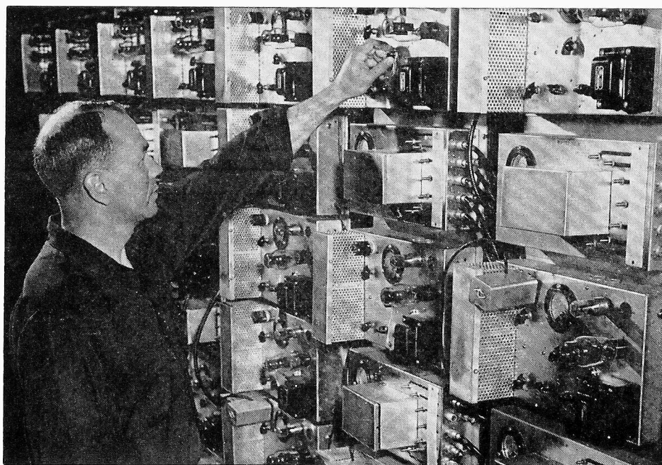
Les Becker adjusts one of the "Gold Room" transmitters.
