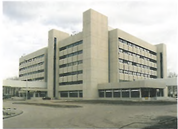
Fig. 2. The building where the circuits will be designed with the help of computers (CAD, Computer-Aided Design).
