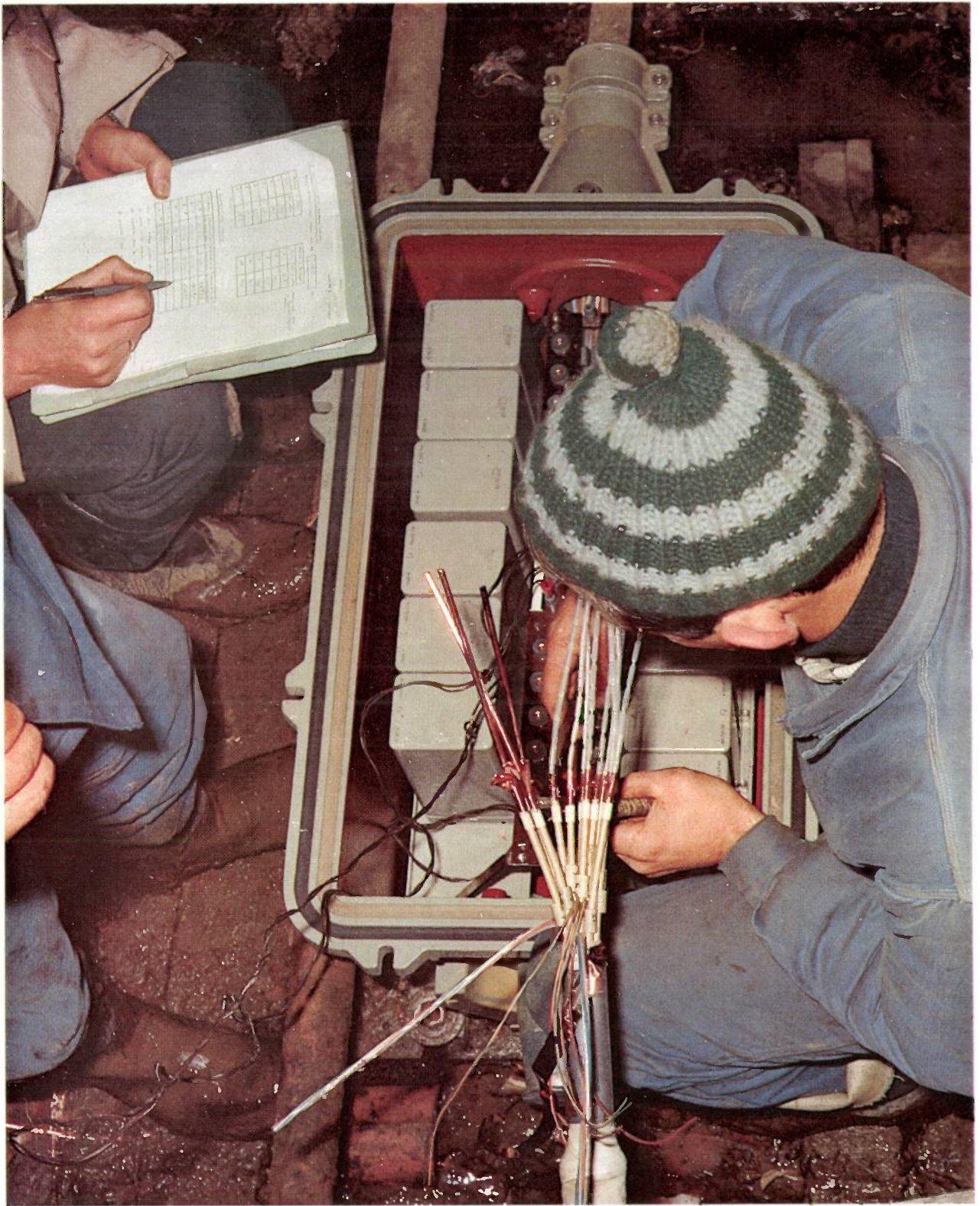
An underground line amplifier (repeater) for 60-MHz cable transmission. The cable contains twelve coaxial cores, each carrying 10 800 telephone conversations in frequency-division multiplex (FDM). A thirteenth core with its amplifier repeater serves as a service channel. These line repeaters are spaced at intervals of 1\frac{1}{2} kilometres (about 1 mile).
