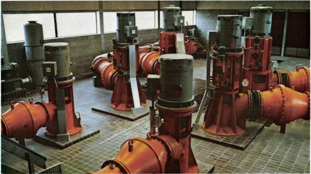
Pumps at the Loerneveen station. The two pumps in the foreground are for filter backwashing, the four at the back for the transport pipeline.
