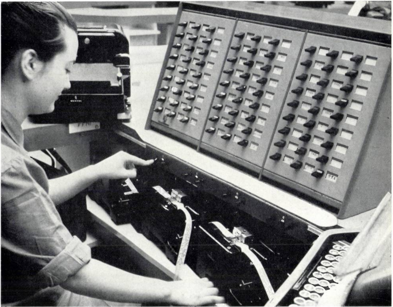
Fig. 6. Operator's position for an exchange based on the arrangement in fig. 5, as adopted in the SITA switching centre in Paris. In front of the operator are four tape transmitters, and above them, the keys that operate them. At the top is a pushbutton panel which is common to all transmitters and has a button for each outgoing route. The reperforators are arranged in two tiers on each side of the operator.
