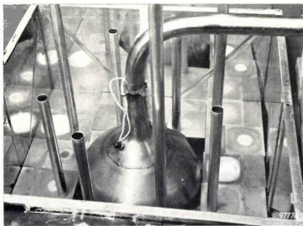
Fig. 5. The reactor vessel in the KEMA reactor I. Of the eight vertical tubes three serve as guides for the control and safety rods; the five shorter tubes each contain a neutron detector. The blocks (partly removed) inside the four walls are of beryllium oxide; together with blocks of graphite outside the walls, they constitute a neutron reflector. The reactor vessel is of stainless steel; it has a capacity of 18 litres and measures 30 cm in diameter. A temperature sensing element is fitted to it.
