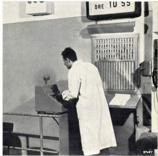
Fig. 4. The stage manager at the Scala has a control desk with a microphone, amplifier and switches; the desk allows him to contact artistes, individually or in groups, via the cables and loudspeakers of the monitoring system, to call them "on stage".
