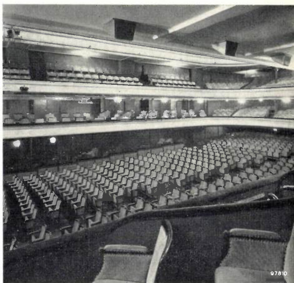
Fig. 15. Auditorium of the Gebouw voor Kunsten en Wetenschappen in The Hague, viewed from a box on the first balcony. Three of the small loudspeakers may be seen along the lower edge of the second balcony.
