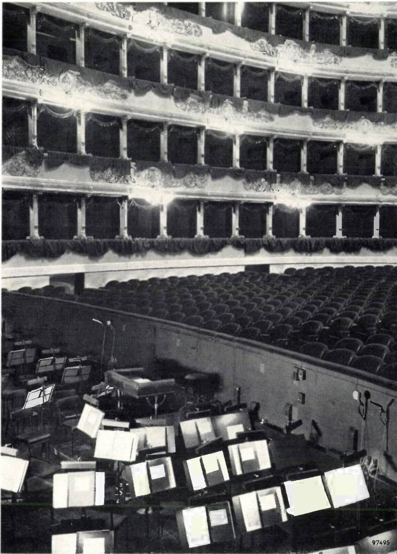
Fig. 2. The auditorium of the Scala theatre, Milan. The acoustics for music are favoured neither by the conventional siting of the orchestra in an orchestra pit, nor by the boxes (only four of the six tiers can be seen in the photograph).
