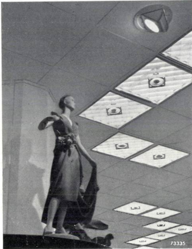
Fig. 7. Department store of Vroom and Dreesmann at Haarlem. The decorating and lighting system is similar to that of Rotterdam ( fig. 6 ), but the ceiling is given a brightly painted surface with a high lighting level. The concentration of attention on the merchandise in this case is in our opinion markedly less.
