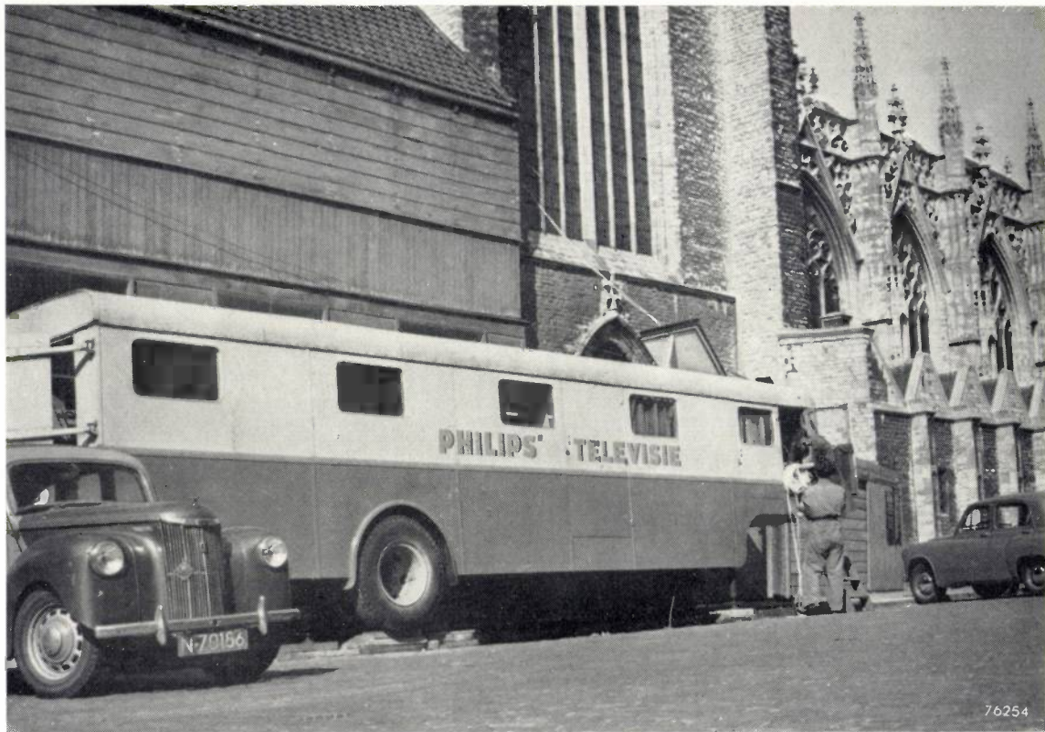
Fig. 2. Trailer housing the 405-625 "line-converter", at the foot of the church-tower in Breda on which a radio-link receiver and two transmitters are installed.
