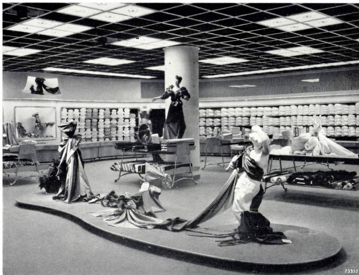
Fig. 6. Part of the department store of Vroom and Dreesmann at Rotterdam. The merchandise is made the centre of interest throughout by local lighting of a high level. The ceiling is painted dark blue. In each quadrangle of the ceiling either a lighting unit, a loudspeaker or a clock can be mounted. The general lighting is effected by means of groups of two 40 W fluorescent lamps with two 68 W incandescent reflector lamps employed as ballasts, each group being inserted in two adjacent quadrangles of the ceiling (in this part of the store double groups are used). As the ceiling itself, lying above the bright metal strips, is almost completely invisible, the architects obtained here an easy method of concealing and at the same time keeping accessible the wiring and plumbing of the store, as well as the ducts for air conditioning. This "Rotterdam ceiling" has since been adopted by a score of department stores in Europe.
