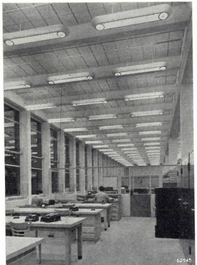
Fig. 10. Room in Philips' head offices at Eindhoven illuminated with lamps in fixtures of the type XA 240 (fig. 9).
