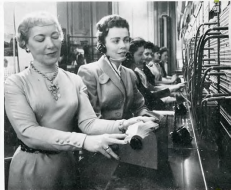
CHIEF OPERATOR KITTY HARRIGAN checks a number with Trixie Olesen, long distance operator at Plant 50's six-position switchboard.
