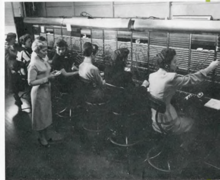
PLANT 50 six-position switchboard. Left to right: Marie Metzler, teletype and Western Union operator, providing relief on switchboard; Ruth Kent, Washington tie-line operator; Arlene Odom, telephone operator; Rose Riotta, telephone operator and relief on teletype and Western Union; Ann Sweeney, long distance operator assistant; Catherine Walsh, telephone operator and relief on teletype and Western Union; Trixie Olesen, long distance operator. Talking with Miss Riotti is Kitty Harrigan, chief operator.
