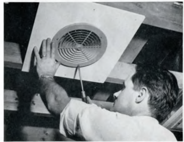
FINISHING THE INSTALLATION of the air supply outlet by screwing in the louvre grille. Five such outlets are provided in Philco's "do-it-yourself" central air-conditioning kit.
