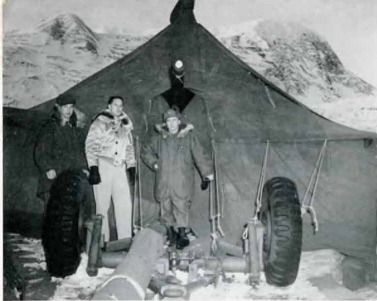
A UNIQUE TYPE of snow cover, to protect anti-aircraft weapons from the ice and snow of Alaska's winters, is shown with its designer (center), Richard Wells, Philco TechRep. The cover consists of three parts, making it capable of being easily transported to and from firing ranges. The first component of the snow cover is a frame made of 3/4-inch salvage pipe which can be quickly reassembled to fit around the gun. An old pyramid tent to which has been added an 18-inch canvas skirt is then placed around the frame. The tent is held upright by a center pole resting on the metal plate of the radar ensemble. The last part of the cover ensemble is a Herman Nelson heater which circulates warm air inside the enclosure. Two modifications of the heater, an electric motor which replaces the gasoline blower and a fuel oil burner instead of the gas burner, reduce the heater's fire hazards. From left to right in the photograph are Lt. Charles H. Sederberg, TechRep Wells, and Pfc. Edwin D. Jones, Det. Btry. C, 867th AAA Bn., at Port of Whittier, Alaska.
