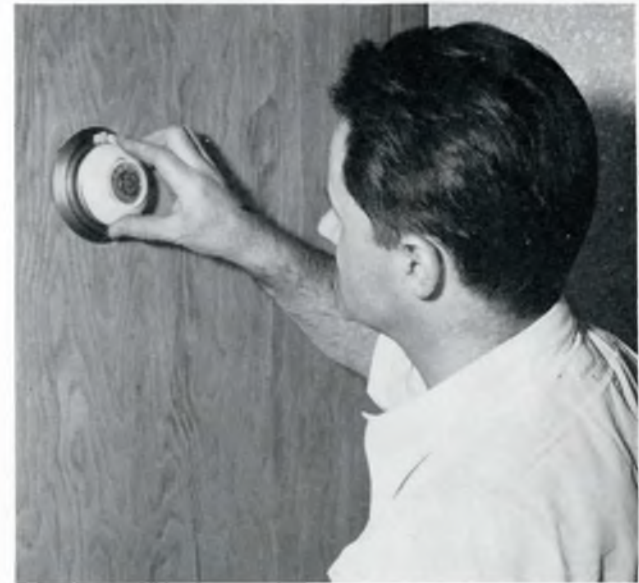
AUTOMATIC THERMOSTAT CONTROL can be placed at any point in the home and automatically keep the temperature at a pre-selected point. Air-conditioning units can also be operated on "fan" only with this control to ventilate home.
