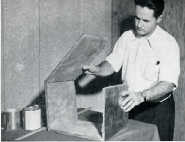
EASE OF ASSEMBLING fiberglass ductwork is illustrated by Ed Poley. Fiberglass is prescored at corners to simplify assembly. Joint sealing tape and compound are provided. Ductwork is aluminum covered to improve further efficiency of insulation.
