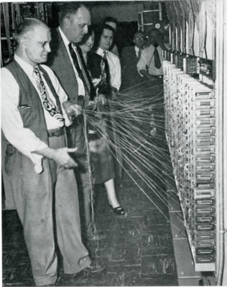
CUTTING OVER from the old to the new switchboard in the new telephone terminal room in the main offices of the Philco Philadelphia plants. Jake Straubline (foreground) is the maintenance man for the telephone company stationed at Philco. Edward Lee, Irene Gumpper, and members of the telephone company staff assist in the ceremonies.
