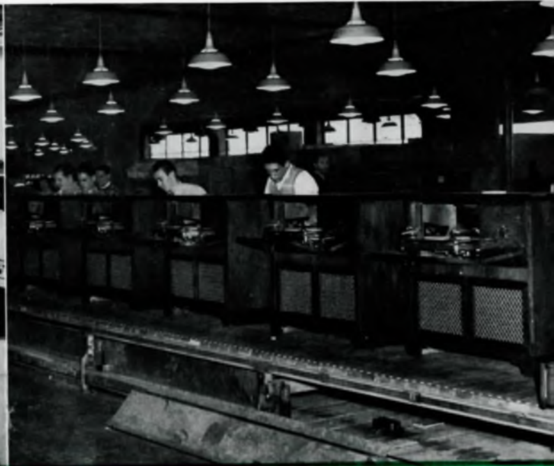
▲ FINAL ASSEMBLY and checking of the Philco 1213 radio-phonograph in Plant 3.
