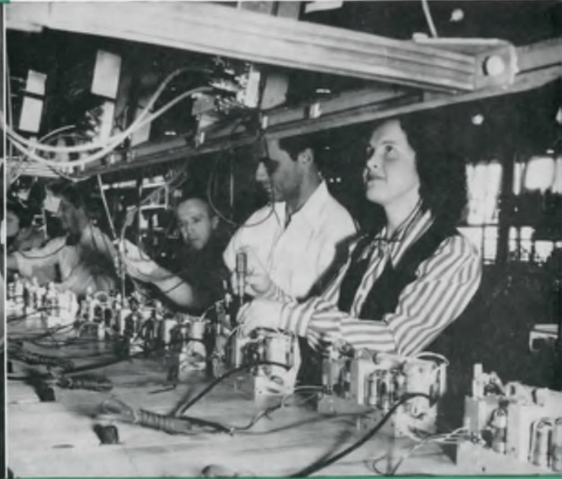
▲ TESTING the Philco 1201 in Plant 3. Frank Henny is the supervisor.
