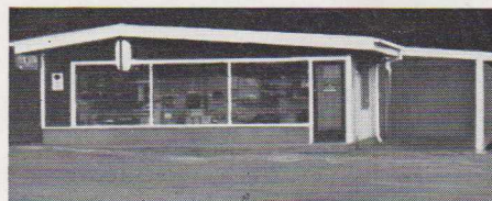
Headquarters of Amalgamated Electronics Limited.
