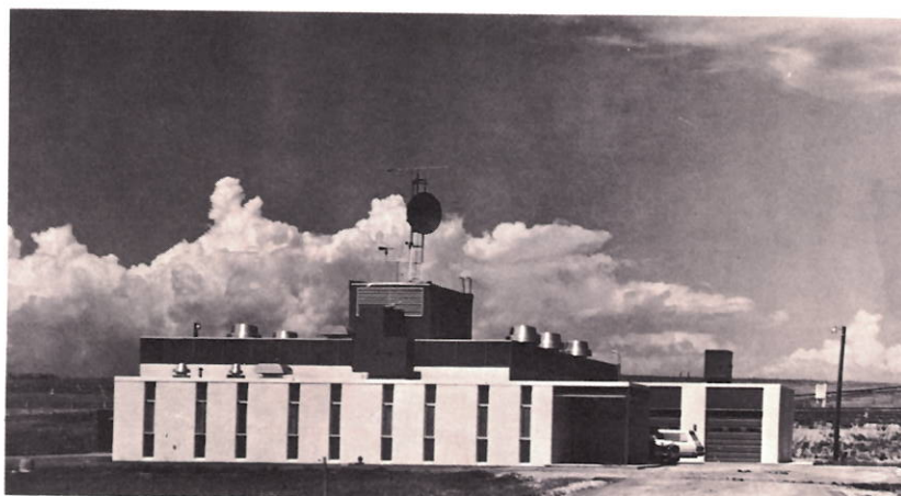
Figure 9—WWV Transmitter Building, Ft. Collins, Colorado.
