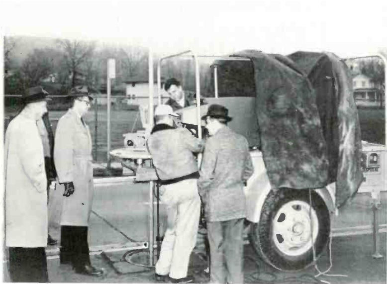
Figure 1 — City of Cincinnati, Ohio Diamond Television System is completely portable. It is mounted on a surplus Army one ton cargo trailer. Shown in operation here, monitor screen shroud cuts down reflections on view screen.
