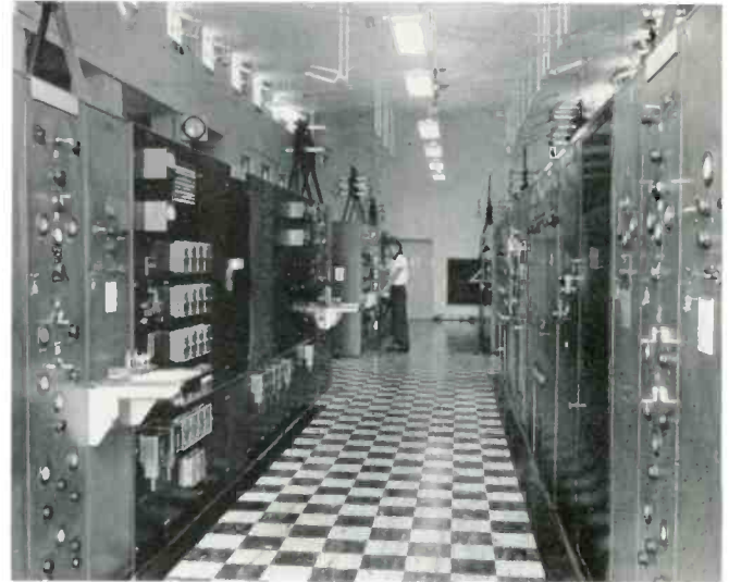
Figure 2 — Main Hall, Transmitter Building #1.
