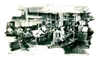
In the Model Shop expert machinists and glass workers fabricate pre-production tube components.
