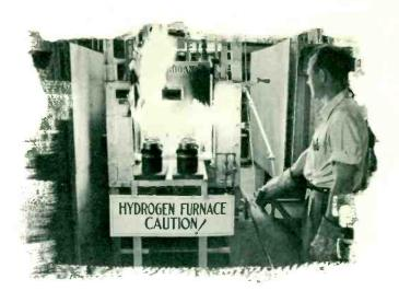
Metal parts are brazed in the intense heat of hydrogen flames.
