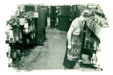
Believe it or not, this is a foundry! The personable young lady in the dainty apron is overseeing the high-vacuum induction casting of copper anodes—a process developed by Machlett Laboratories and unique to Machlett Laboratories.
