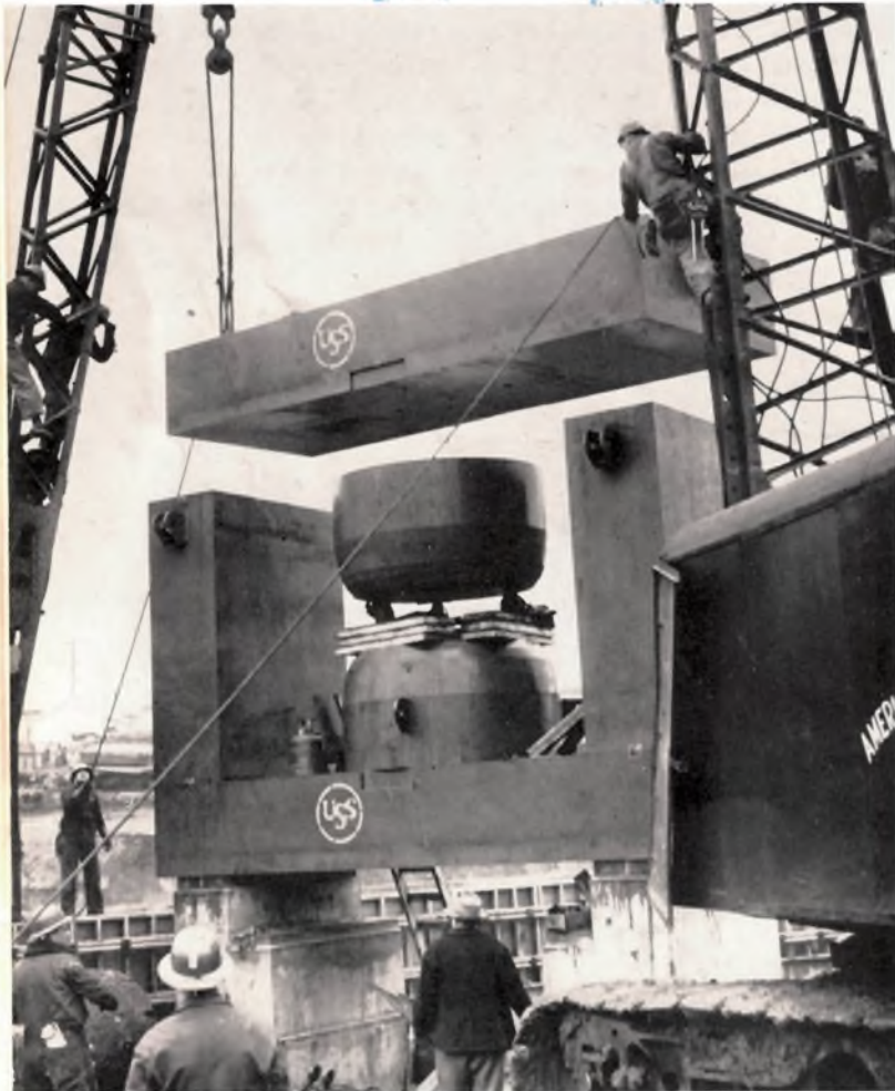
Figure 1—Placing of the 67-ton top member on the 250-ton magnet of the Collins cyclotron.
