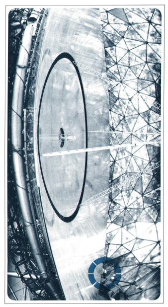
Fig. 6. The 120-foot anterna at Lincoln Laboratory's Haystack Microwave Research Facility. Notice the man at the bottom. Haystack is one of several radar and radio astronomy facilities which use hydrogen masers as frequency standards.
