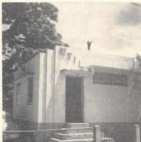
WTIL in Mayaguez, Puerto Rico has as modern a transmitter building as you will find anywhere. The order for the Gates equipment was negotiated in 1950 by our Sales Manager, Larry Cervone and Mr. Patricio R. Fermainitt, Gen. Mgr. of WTIL.
