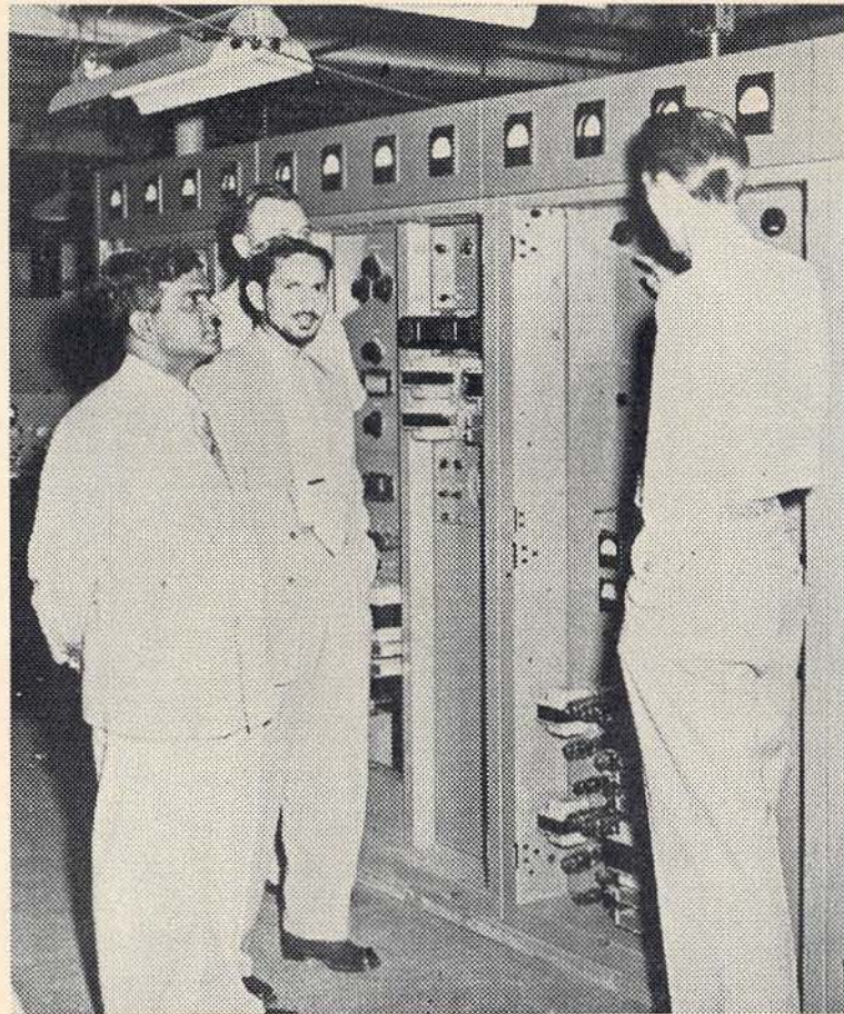
John D'Cruz and Abdul Rauf, from left to right, are inspecting a Gates 5-kilowatt television transmitter. Gene Hildebrandt of the television department can be seen behind Mr. Rauf and television engineer Bill Parker is making the explanation.
