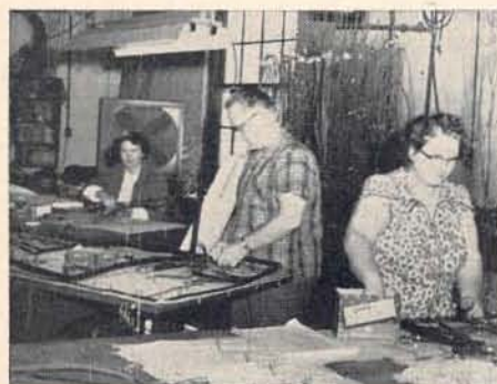
Rose Ballow, Clarence Kinder and Katherine Dorsey are all working on cables for 250 GY Transmitters. A small portion of wire stock can be seen hanging on racks in background.
