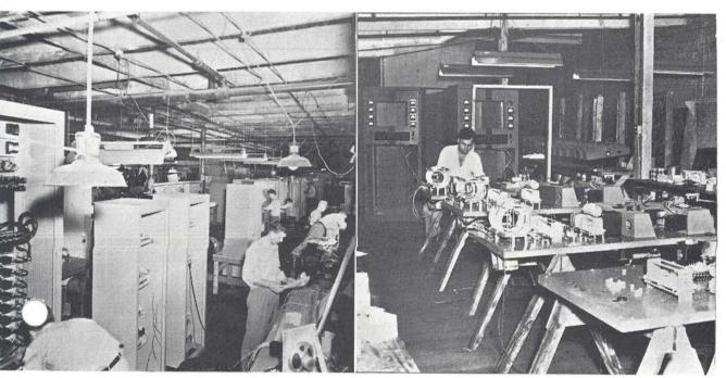
One of the assembly lines of speech cabinets and 1 KW transmitters. (Left)
