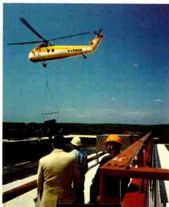
New General Electric Headquarters, well on its way to completion amid meticulously landscaped hillsides with terraced rock walls, already includes finished offices, as previewed at left. Helicopters were used to lower air conditioning units into place on the buildings' rooftops. Integrated modular ceiling units provide heat and air conditioning outlets as well as lighting.
