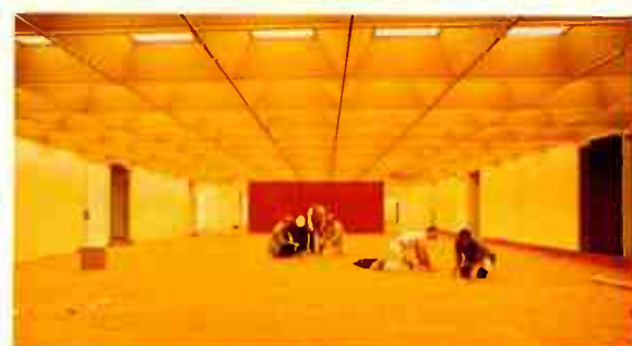
New General Electric Headquarters, well on its way to completion amid meticulously landscaped hillsides with terraced rock walls, already includes finished offices, as previewed at left. Helicopters were used to lower air conditioning units into place on the buildings' rooftops. Integrated modular ceiling units provide heat and air conditioning outlets as well as lighting.
