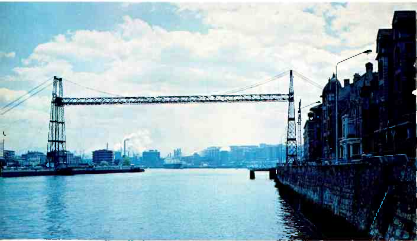
Regional landmark for GEE people in Bilbao is the "hanging" bridge over the Nervion River. Busy harbor traffic makes cantilever or drawbridge impractical. Solution: pedestrians and cars are carried on barge-like above-water platform suspended from rollers on bridge superstructure. Below: big 541-megawatt turbine-generator at Santurce thermal plant represents joint manufacture by GE-USA and Española.
