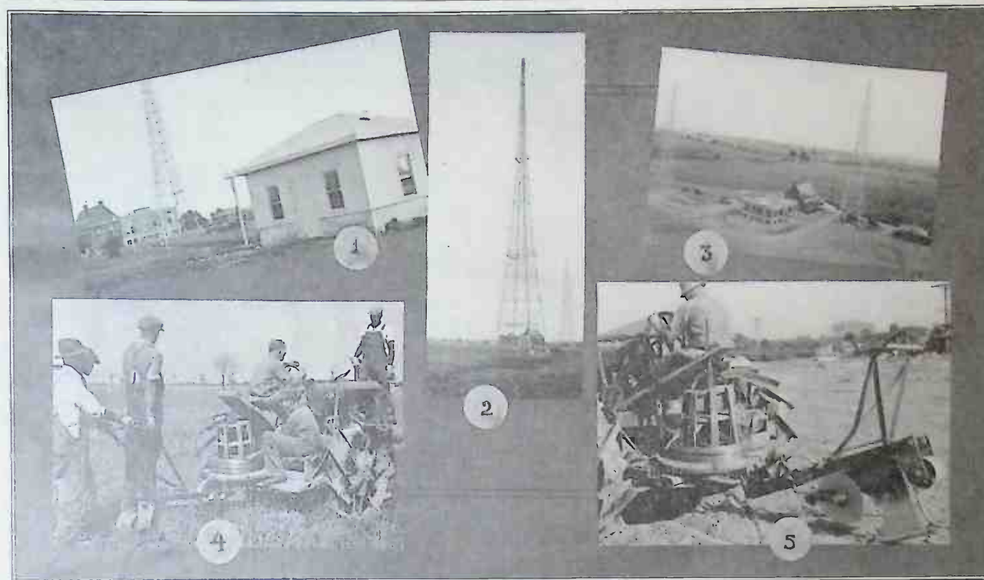
1. Coupling house at WLW station, Mason, Ohio, used for equipment for coupling transmission line to antenna. 2. One of the 300-foot towers of the new WLW station. These towers are constructed of galvanized steel. 3. Aerial view of station at Mason, Ohio, with transmission buildings for WLW and WSAI. The towers shown in this photograph are used by WSAI. 4. The crew which "sowed" the copper wire between the two great towers of WLW. 5. Machine used in "sowing" copper wire; this machine ploughs the ground, lays the wire in the furrow, and covers wire over with earth.
