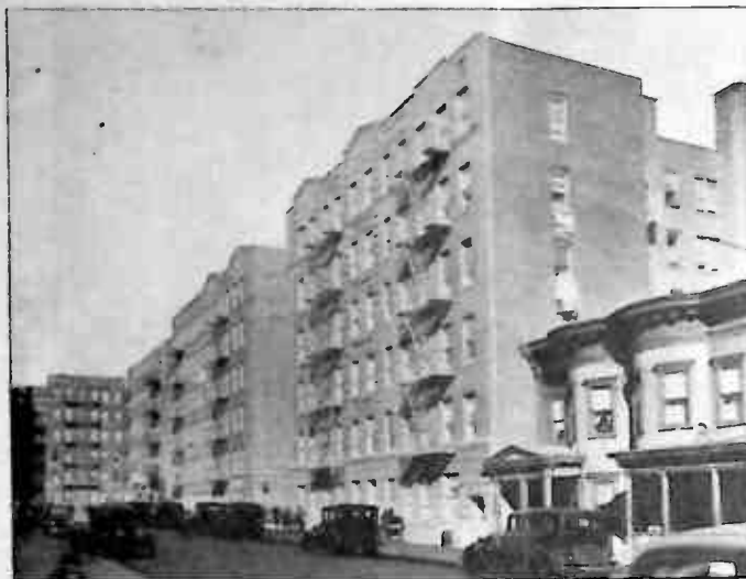
Above: Is a beautiful New York Apartment house at 2160 Clinton Ave. 110 Crosley Shelvador refrigerators were installed here.
