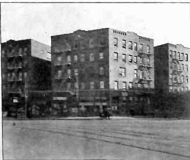
Left: Here is the attractive apartment building at 1210 Westchester, New York City, where 102 Crosley Electric Refrigerators were installed.
