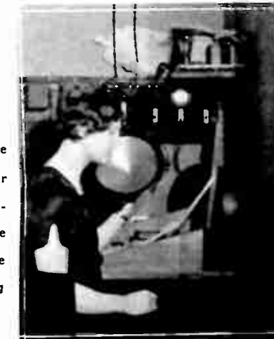
BOBBIN WINDING OPERATION. On each arm of the armature is a small bobbin. Just as the armature is the most important part of the Dynahone, the bobbin is the most important unit of the armature. The bobbins carry the wiggles of signal current which are converted into sound.
