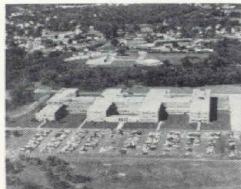
Airplane view of the new General Radio Plant.
