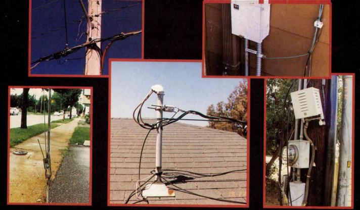
Top left: The CATV system is just a few inches from street light power. Top right: The NEC does not permit grounding to a flexible conduit. Bottom left: A missing down guy guard presents a hazard to pedestrians. Bottom center: The
