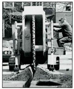
A rock saw is used by McCourt Cable Systems as part of the CATV construction process that reduced underground building time in Boston nearly 50 percent.
