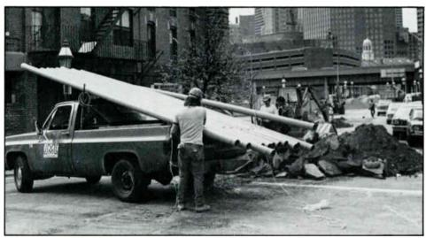
Before introducing the MBI construction process in Boston, McCourt Cable Systems employed the traditional building method of digging deep, wide trenches, emplacing short conduits, then pulling the cable through the ducts.
