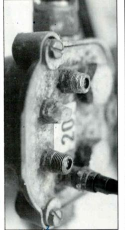
Corroded tap fittings prevent good ground contact while broken fittings prevent installation of terminators.
