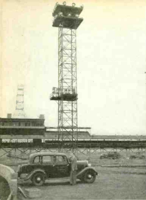
FIG. 6. THE LOUDSPEAKER INSTALLATION AT ROOSEVELT RACEWAYS. NINETEEN 1000-WATT UNITS AT THE TOP OF THE TOWER PROVIDE GENERAL COVERAGE, WHILE TWELVE SMALLER UNITS, FURTHER DOWN, COVER THE GRANDSTAND DIRECTLY IN FRONT.
