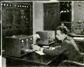
Frequency monitoring units on desk at WHN, and station speech input equipment at right.
