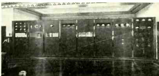
Western Electric 50KW Transmitter at WJR.
