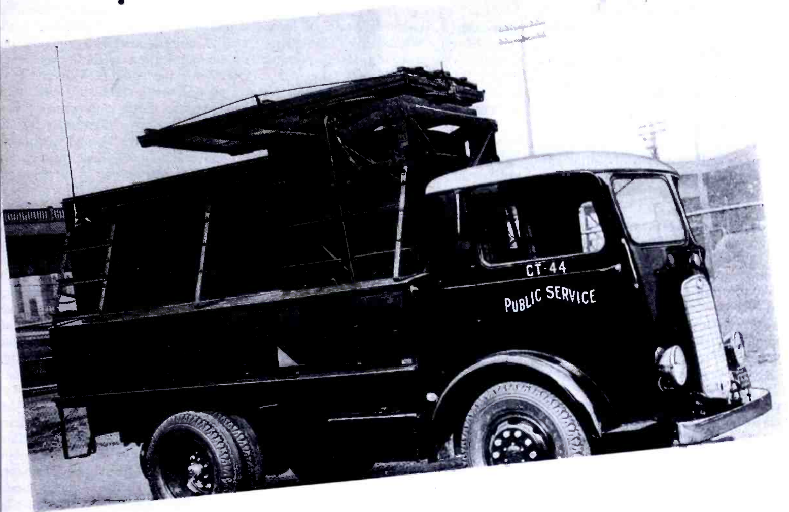
Typical communications-equipped power company service truck.
