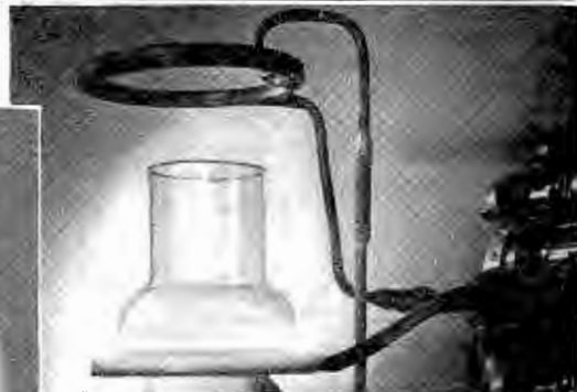
The use of R. F. heat in making glass to metal seals simplifies and speeds many such sealing operations
