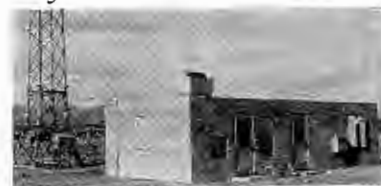
Right, finished transmitter building at South Pacific project.
