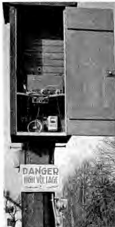
Figure 12 F-M receiver mounted atop a mountain and in continuous operation that serves as a reliable receiving station for the New Hampshire state police.
