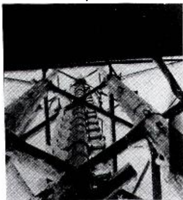
Above: Fig. 41. Showing ice formation on antenna. Above, right: Fig. 42. Lightning striking Empire State Building.
