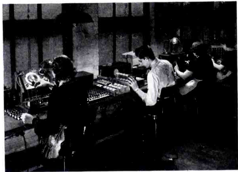
Fig. 1. Component parts being individually pre-tested before going into receivers.
