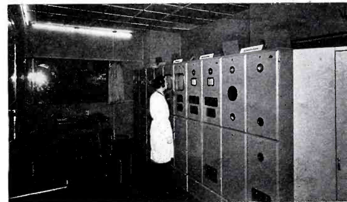
Fig. 9. (Above) Synchronizing apparatus, mixer and controls of Safar television cameras.
