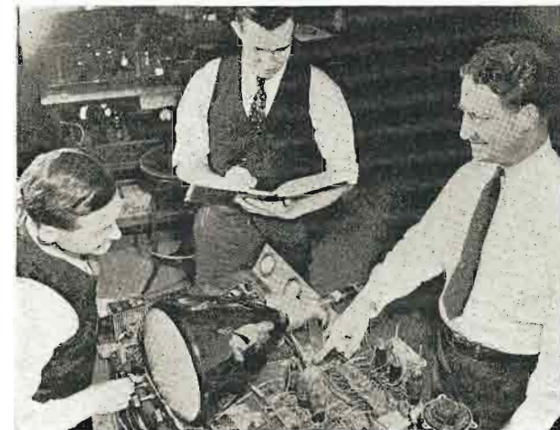
Above: Fig. 7. A 12" cathode-ray tube being subjected to factory tests. RCA photo.
