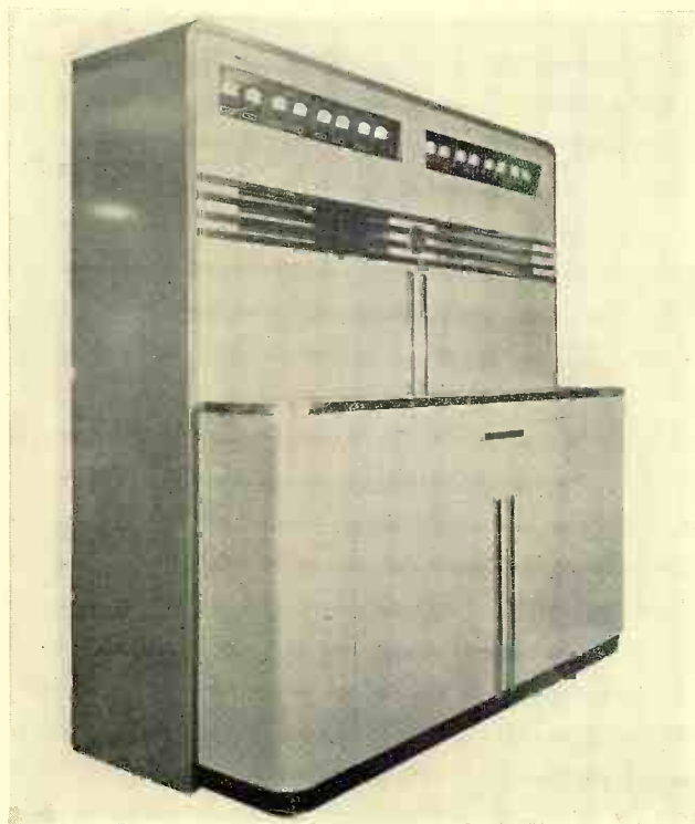
Fig. 4. The RCA 1000-watt picture transmitter. It is believed that the power of this transmitter, with a suitable antenna, is sufficient to render a satisfactory service over a reasonable area. It conforms with the RMA standards.
