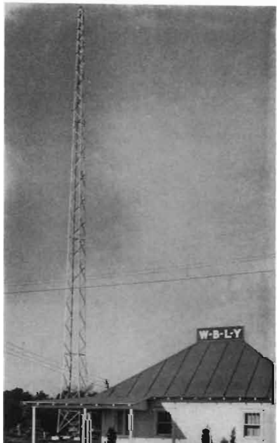
WBLY, Lima, Ohio. This self-supporting type Ideco antenna is 154 feet high.
