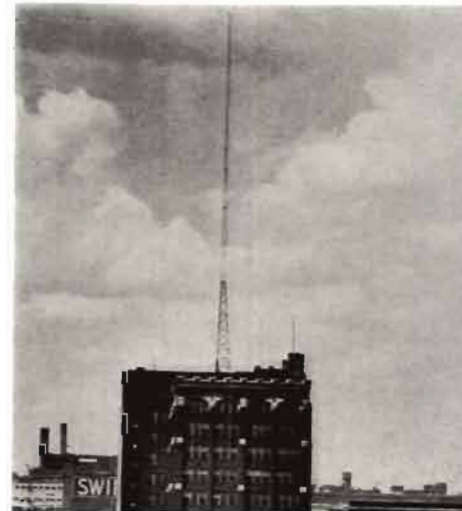
The 231-foot Truscon self-supporting radio tower at WAAF, Chicago, Illinois.
