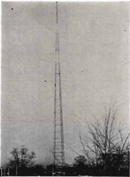
WMAS, Springfield, Mass. This 350-foot radiator was built by the Blaw-Knox Co.
