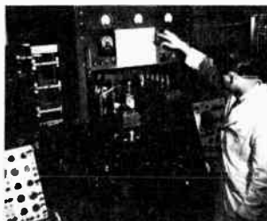
6 MILLION WATT PULSE MODULATOR
