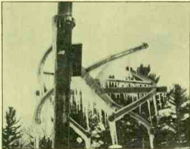
Figure 7 - BFM Antenna with Icing
