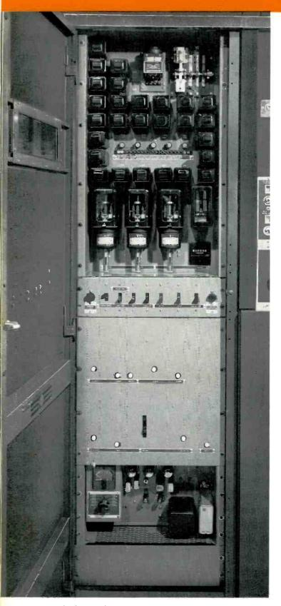
Control calcinet with door open showing au≻iliary switches, breakers, overload and auxiliary relays. Overload inditating ights for all TT-25DH «incuits are g⊪owped on strip that tan be seen through window when door is closed.
