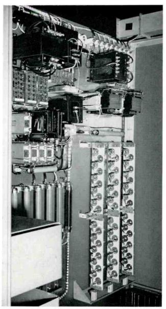
Photo of the rectifier panel showing completely siliconized power supplies. At the lower right are the silicon diodes that make up the 4800-volt rectifier thus eliminating all mercury-vapor rectifiers.
