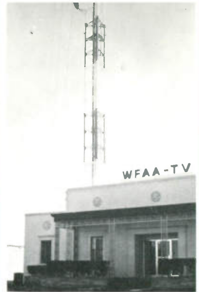
WFAA, Dallas, Texas. FM Stereo to Cedar Hill (18 airmiles) to TV-FM site. Using 7 GHz. Passive Reflector.
