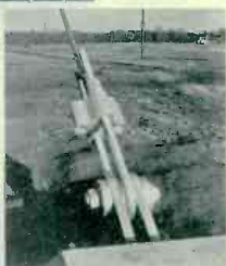
Typical guy anchor.
