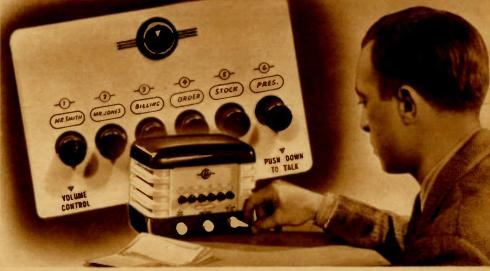
MASTER STATION AND ONE REMOTE STATION WITH TUBES
